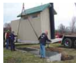
Offload by Crane
